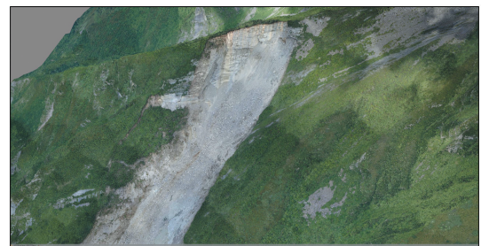
(a) 茂县新磨村右侧变形体
